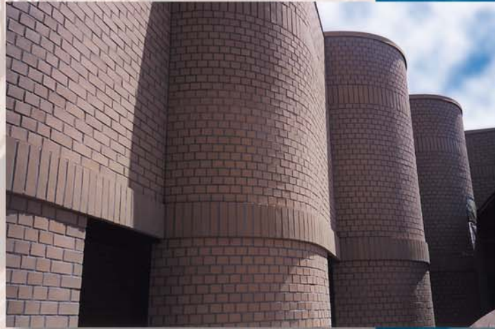
Custom Color, Medical Building, Riverside, California
