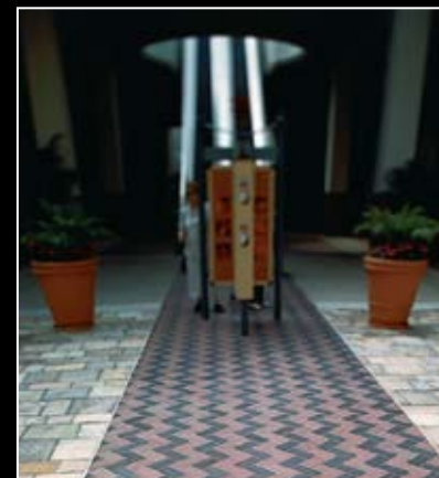
Fashion Valley Mall – San Diego, California Rose Blend Wirecut – 1/2'' \times 3\frac{5}{8}'' \times 7\frac{5}{8}'' and Dark Ironspot Wirecut texture – 1/2'' \times 3\frac{5}{8}'' \times 7\frac{5}{8}''
