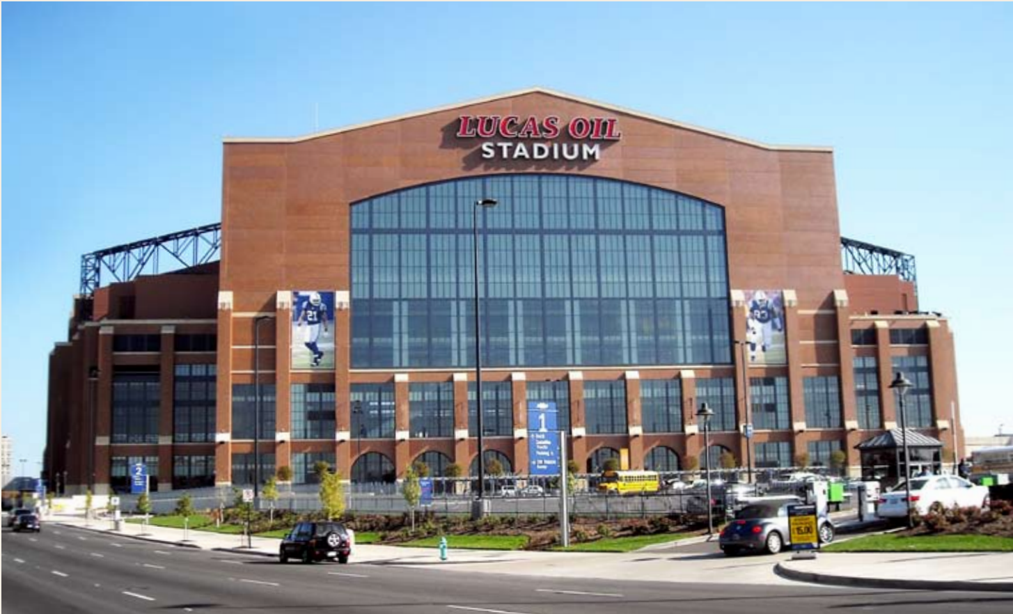
Lucas Oil Stadium – Indianapolis, Indiana Thin Brick
