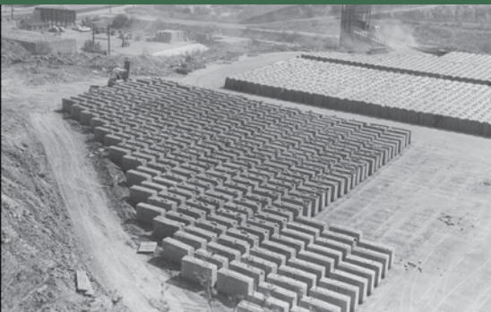
Monterey Park Plant 1950
