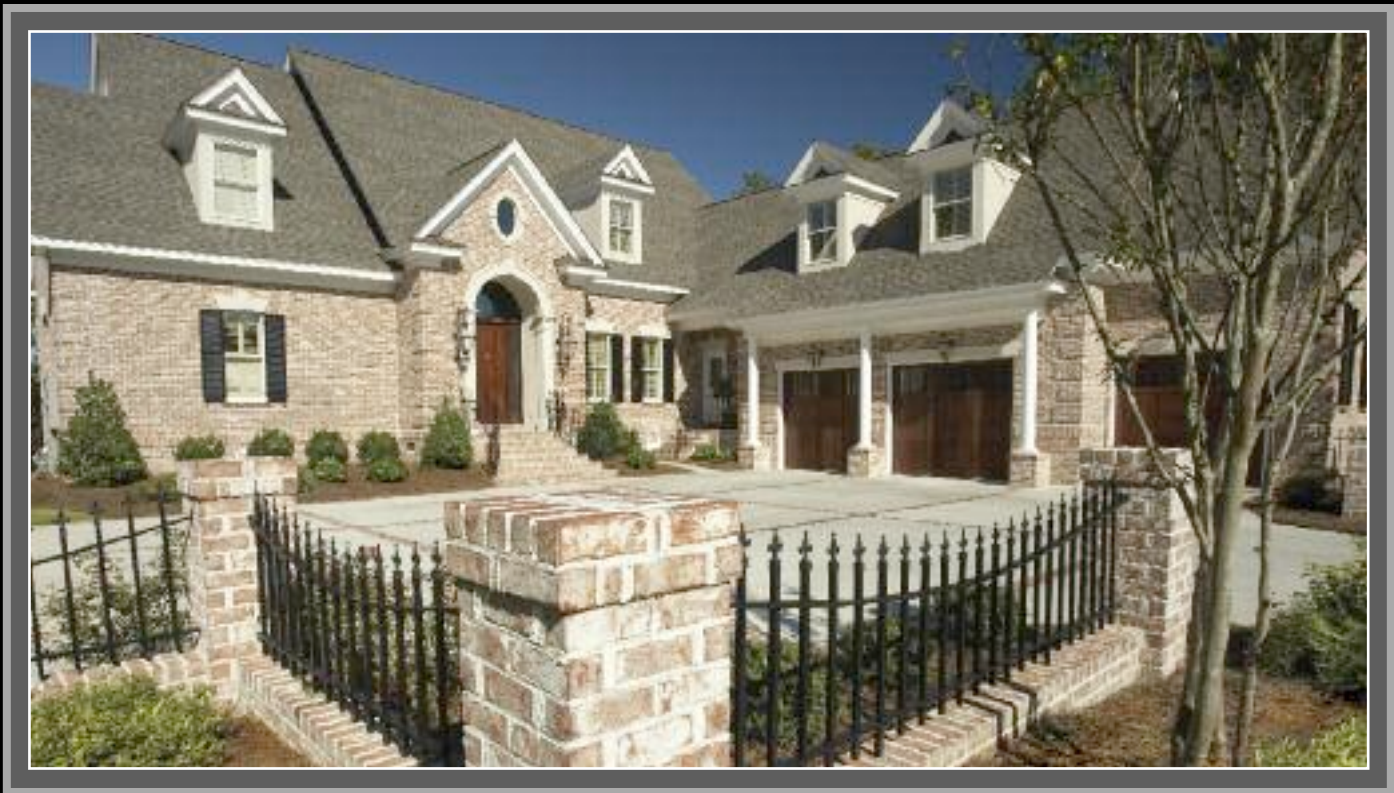
Private Residence • Sierra Queens
