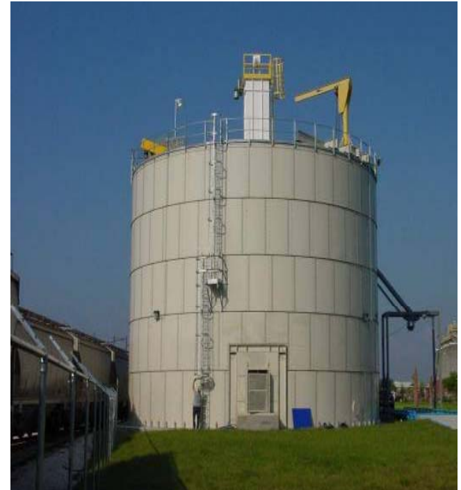
Fly Ash Distribution Terminal, Riviera Beach, Florida
