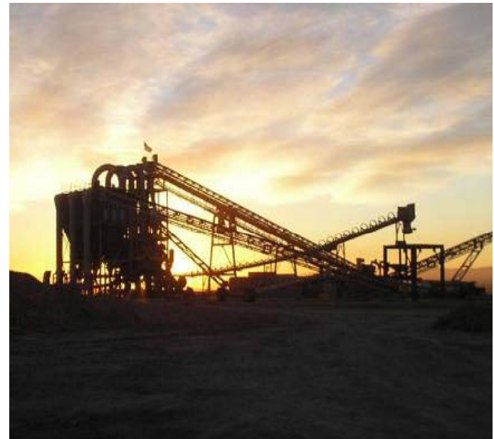
Coal Recovery Facility (Dry Technology) Wellington, Utah
