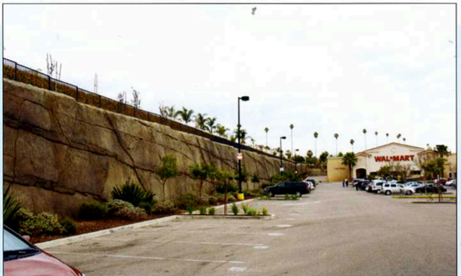
The finished product provided engineered ground support and attractive architectural treatment.
