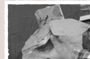
PHOTO 3 - Application of mortar onto Natural Thinstone Veneer.
