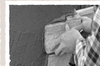
PHOTO 4 - Application of Natural Thinstone Veneer.
